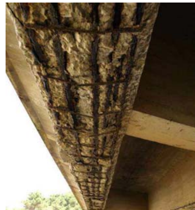
Figure 10. Corrosion in beam 1
