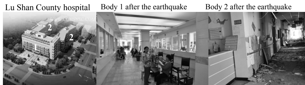
Figure 1. The Lu Shan Hospital: The body 1 is base isolated; the two bodies 2 have traditional foundations.
